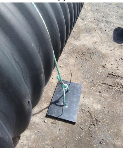
This is an indicative photo to show the placement of the of the pads and the tightness of the rope. It is not an actual install as there is no trench or compacted basecourse shown.
